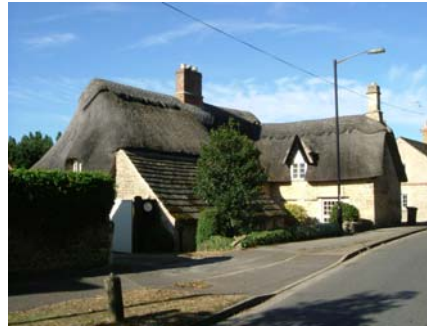
Lower quality rubble stone and rough dressed quoins with timber lintels
