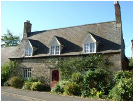
Lower quality rubble stone and rough dressed quoins with timber lintels
