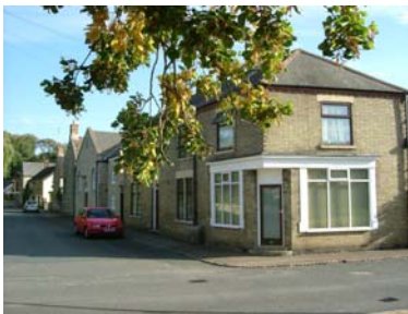
Former shop to Church Hill
