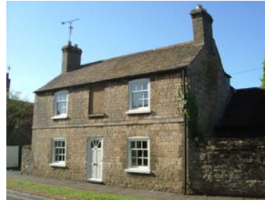
Squared rubble stone and dressed stone quoins, stone lintels (Collweston and slate roofs)
