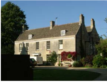
Squared rubble stone and dressed stone quoins, stone lintels (Collweston and slate roofs)
