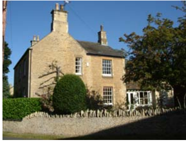
Squared rubble stone and dressed stone quoins, stone lintels (Collweston and slate roofs)
